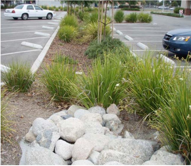
Landscaped island with a bioswale to filter run-off from the parking lot.
