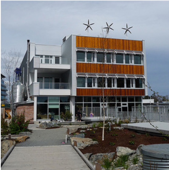
Small wind turbines on the roof of an office building.
