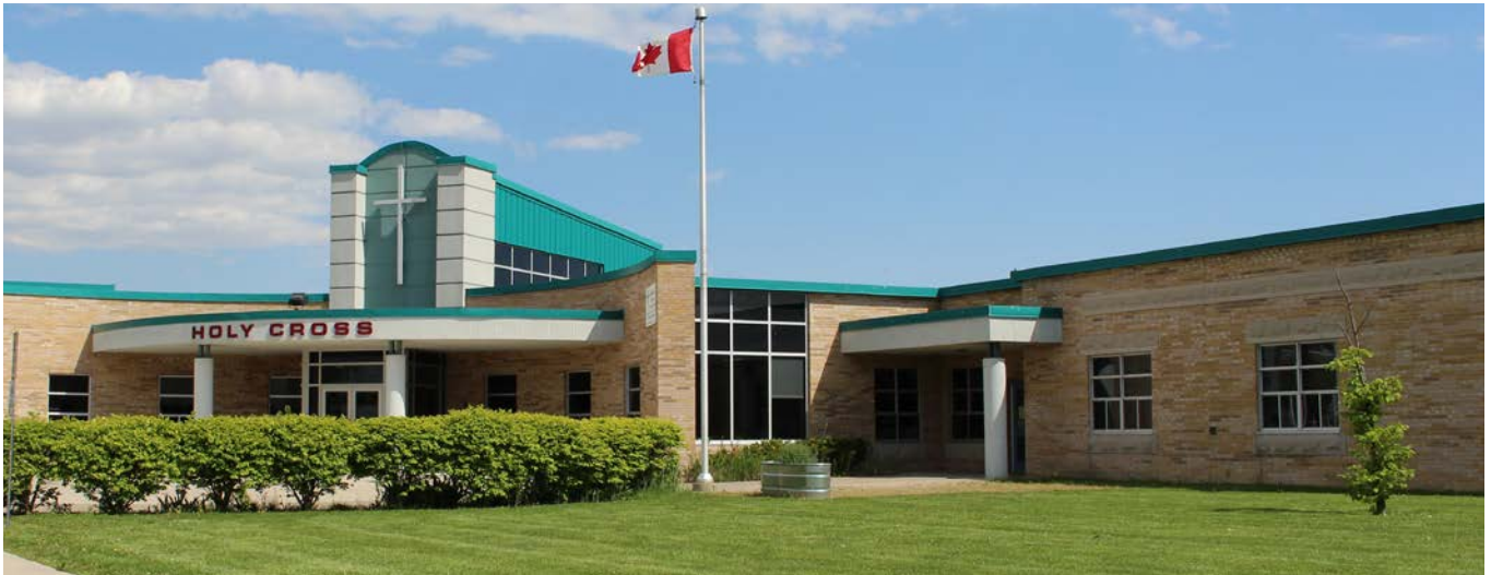
Elementary school with articulated entrance features.
