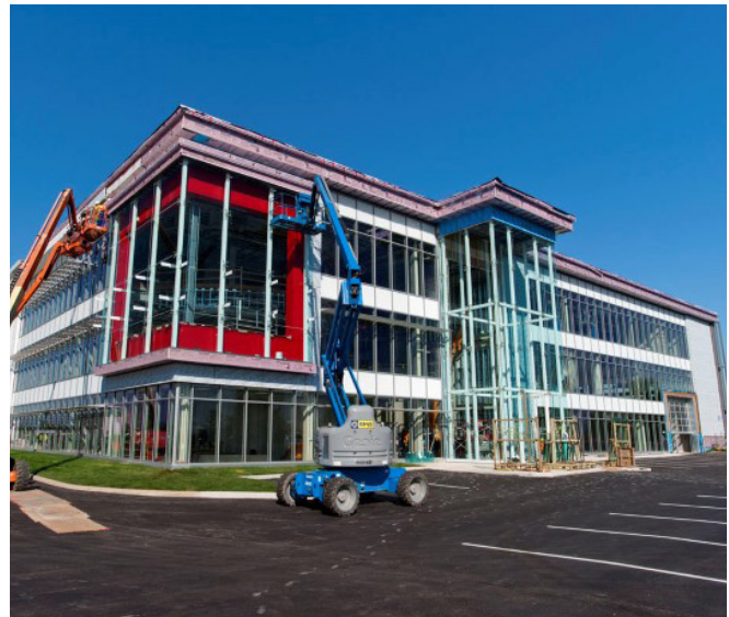
Construction of an employment office building.
