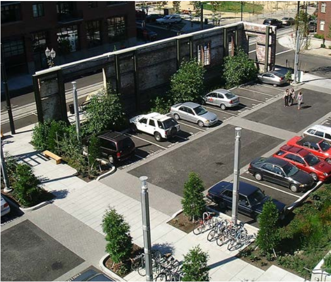
Parking lot with smaller courts, plantings, and decorative paving.
