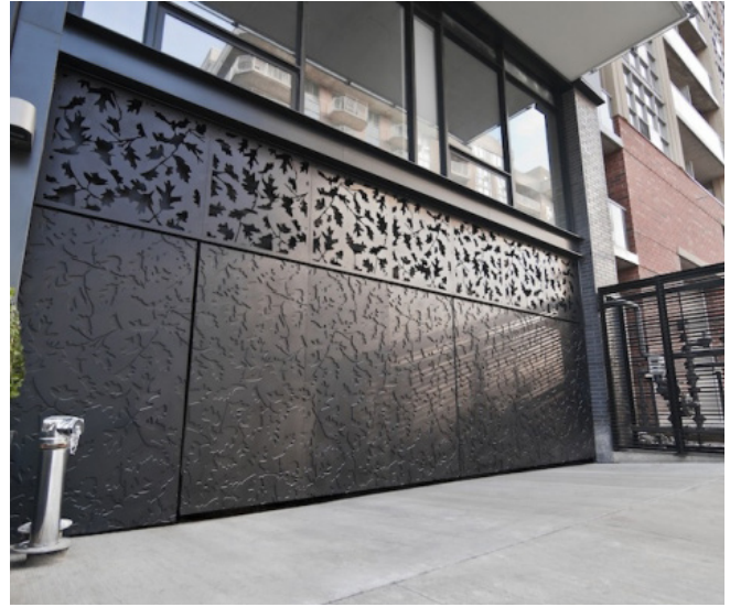
Underground parking garage access screened by decorative door.
