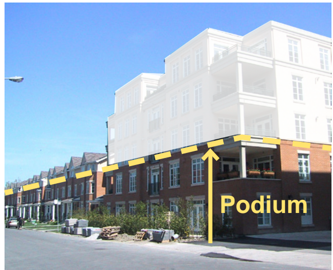
The height of the podium on the mid-rise building should match the adjacent dwellings.
