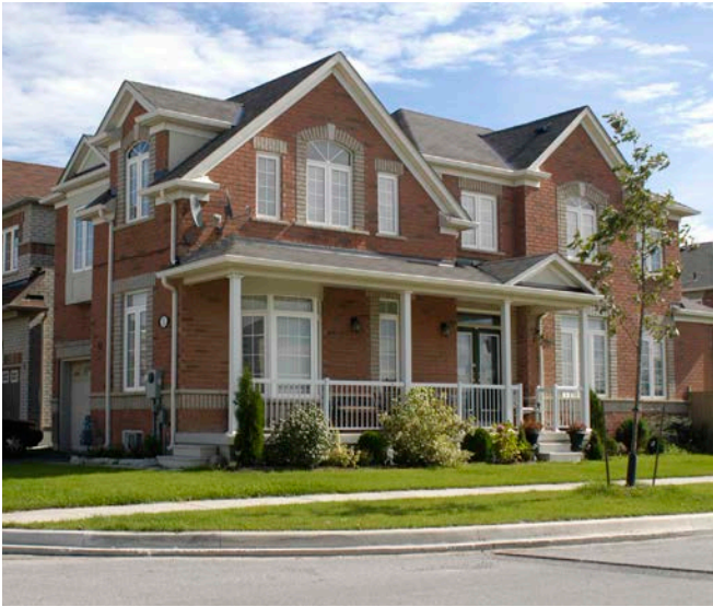
Single detached dwelling with upgraded side elevation.
