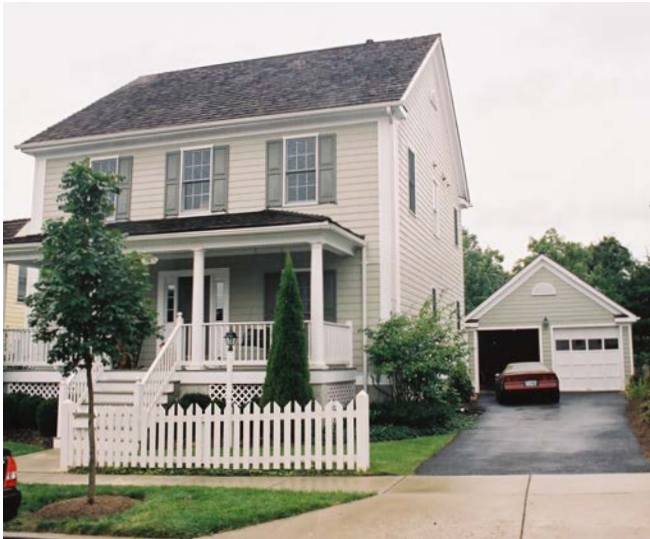
Detached garage located in the rear yard.
