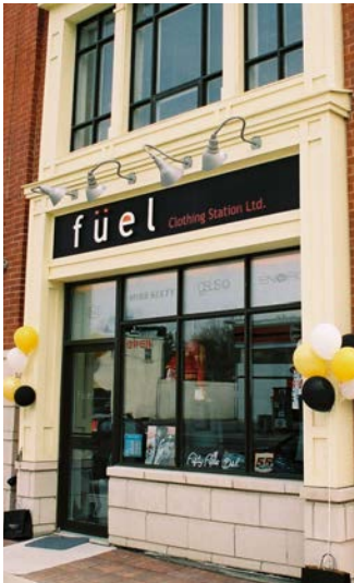
Lighting is directed at the sign and complements the design of the building.
