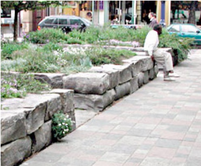
Light coloured pavers assist with the reduction of the urban heat island effect.
