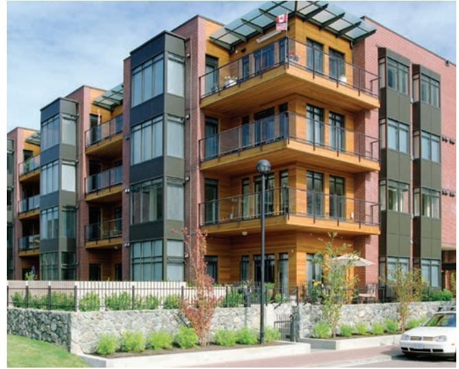
Windows and balconies included on all elevations of the building.
