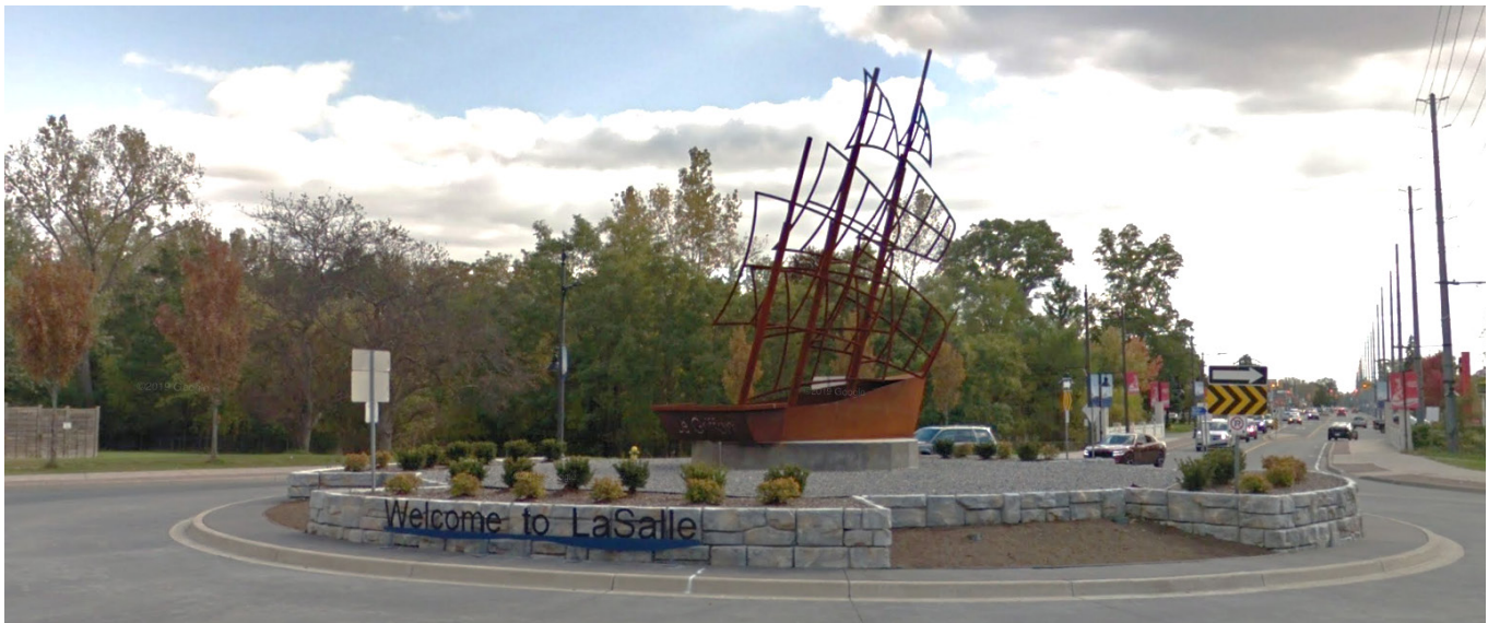
Arterial Road with a roundabout and gateway feature.
