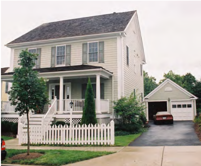
Detached garage located in the rear yard.
