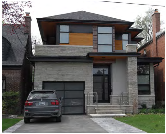
Example of a mix of building materials on the facade of a dwelling.
