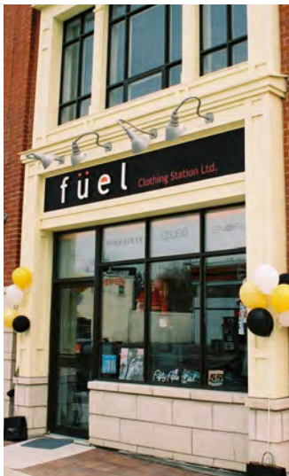
Lighting is directed at the sign and complements the design of the building.
