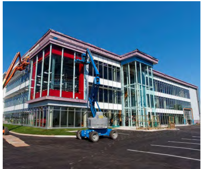
Construction of an employment office building.
