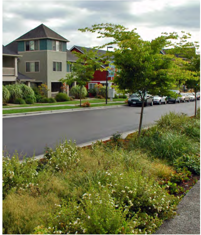
Local Road with a bioswale in the right-of-way to assist with run-off and infiltration.
