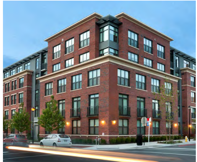
Example of a 5 storey residential building.
