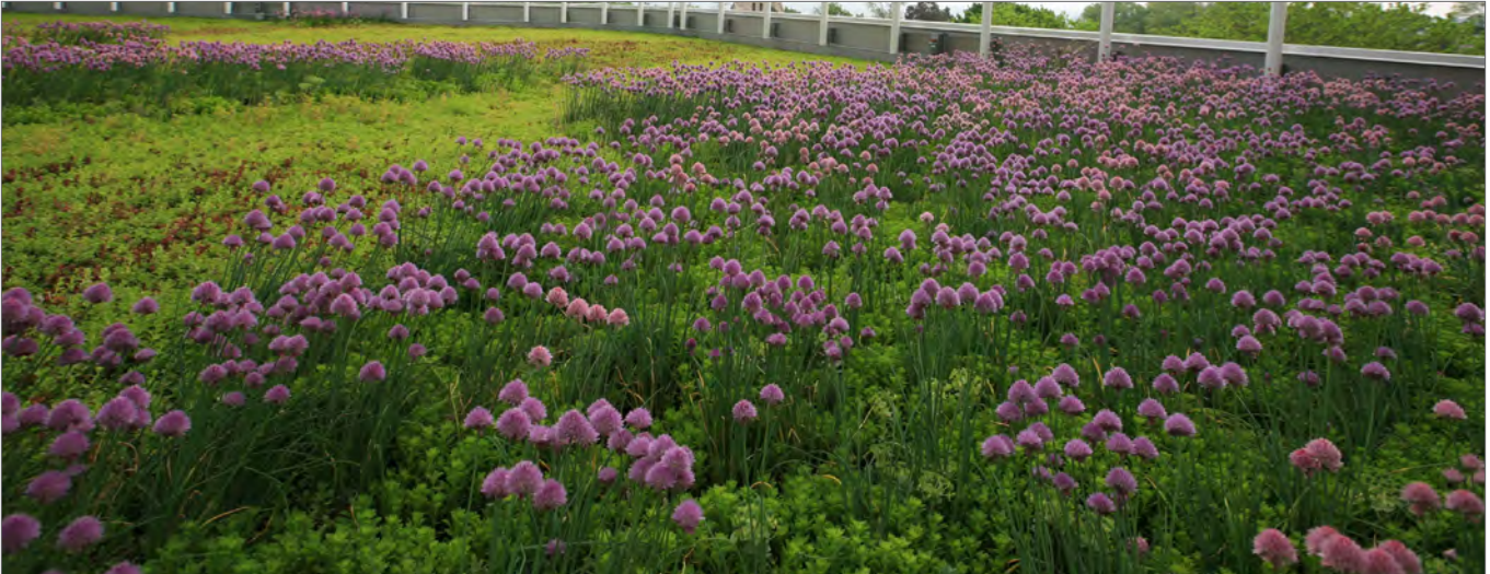
Green roofs reduce surface run-off on buildings.
