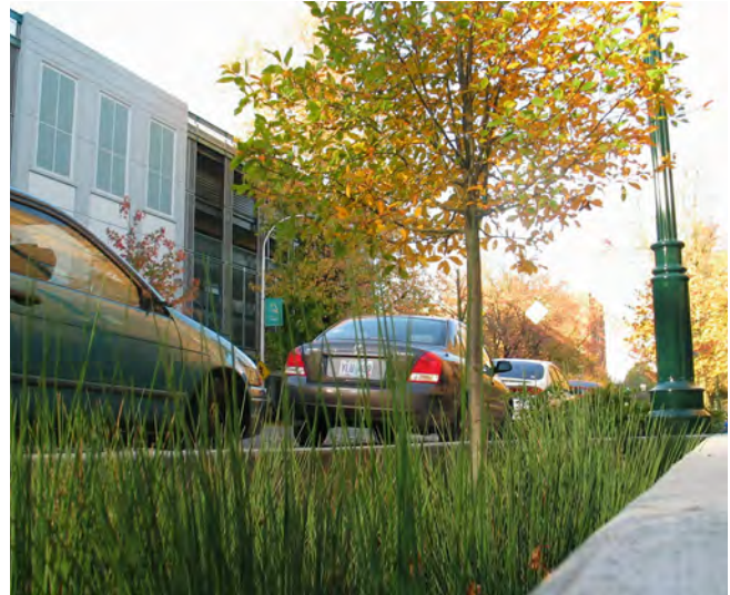
Bioretention planters assist with street greening and have stormwater management benefit.
