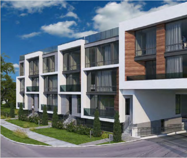
Low-rise building with inset balconies and entrances along the street.
