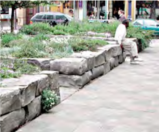
Light coloured pavers assist with the reduction of the urban heat island effect.
