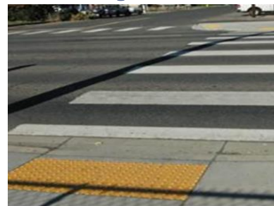
tactile walking surface indicators
